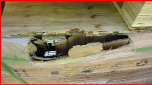
Pallet wear and tear or damaged modules
